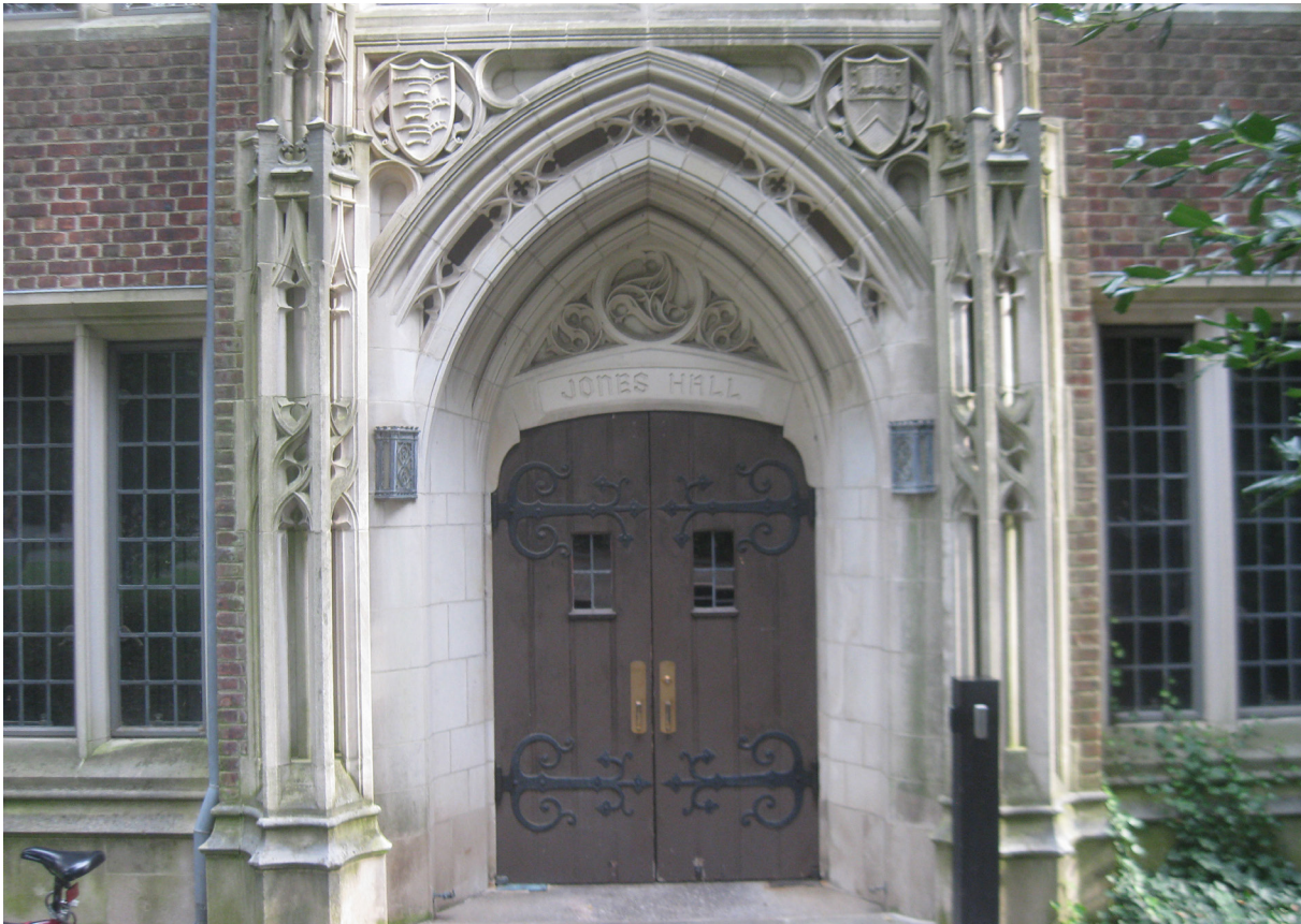
Jones Hall September 2016
